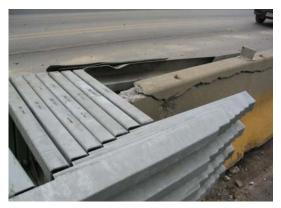
This was an angled impact. A significant object on the Tractor/trailer caught enough of the attenuator to collapse it fully then break the concrete barrier. The speed was probably not excessive so the cylinder did not provide full stopping force but the energy of the Tractor/trailer bottomed out the unit and cracked the barrier wall.
