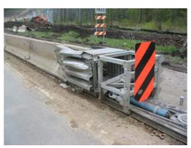
5-25-05 - 2nd Incident – Serial #104 Hit 2<sup>nd</sup> time same day after reset Frontal Impact – Collapse – full No Injuries Part Required – replace unit Repair cost part and labor - \$13,500.00 Vehicle – Tractor/trailer Posted speed – 40
