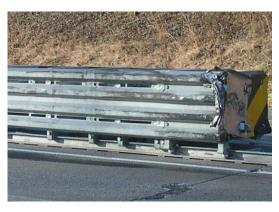
Side view of above incident You can see a piece of the tool box left on the attenuator on the top picture and the tire marks down the side on this picture. The corner was caught and the collapse started. We are coming to the conclusion that truck drivers are able to steer off of our unit. The unit was still structurally sound and ready for further collapse.
