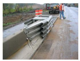
Incident above Shows how the panels nest without being stressed.
